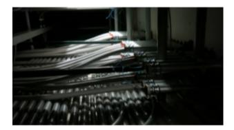
Figure 4 The design choice to use pre-assembled cabling (TC Cable, as pictured) instead of in-house assembled cabling to provide the 24,000 linear feet of electrical cable required to connect Trinity resulted in an estimated \$1M project cost savings.
